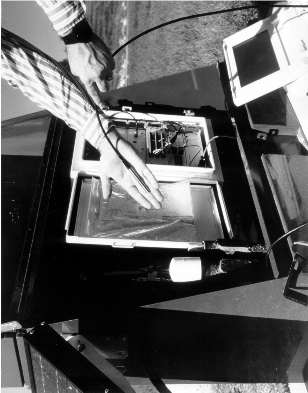
Figure D-2. Remote monitor unit in protective structure showing solar panel, pressure transducer, and portable computer
